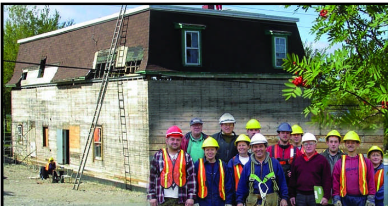
Front from left; Billy Lucas(carpenter apprentice), Penny Cooke-Alexander & Bertha White(labourers), Melvin White(carpenter foreman), Ben Alexander(engineer), Gerard King & Judy Doucette(labourers). Back from left; Adolphe Lucas(carpenter), Leonard Young(project manager), Jeremy Lee(carpenter), Sheldon Lucas(carpenter apprentice), Gregory Young & Joshua Duval(labourers).
